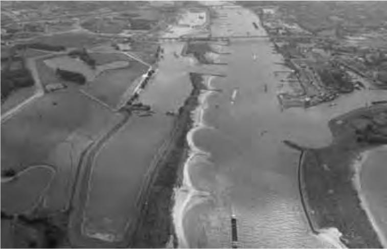
Figure 18. Creating room for the river by cutting a new channel at Nijmegen
