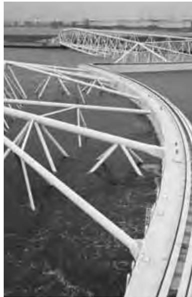
Figure 16. The tubes of the gate are filled with water to immerse the gates into the river canal, erecting the sea wall (Image source: <https://beeldbank.rws.nl>, Rijkswaterstaat)
