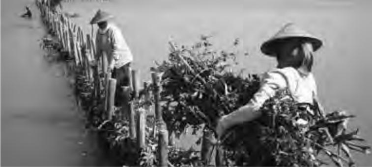
*Figure 2. Building of the semi-permeable wooden dam to recover the mangroves at Demak, Indonesia (Image source: photo by Nanang Sujana for Wetlands International, Building with Nature in Demak, Indonesia)*
