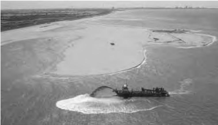
*Figure 3. Sand dredging the Sand Motor*
