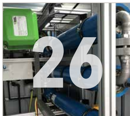
BLUETEC on the rise thanks to Forward Osmosis
